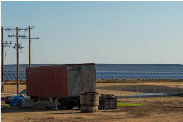
Northfield, Minnesota, USA Solar Garden
