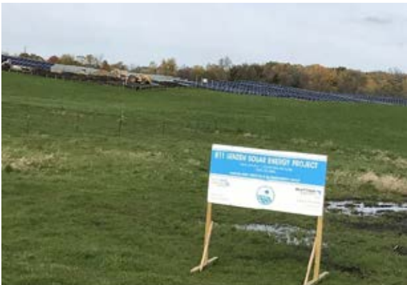
Watertown, Minnesota, USA Solar Garden
